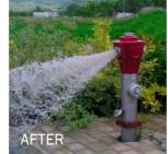
The final pipe flushing is done through hydrants and drains. At end lines the air-water mixture is flushed out through house connections.
