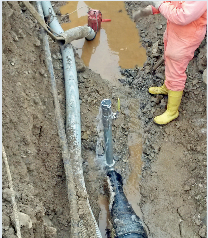
Figure 3: Starting point with water connection point
