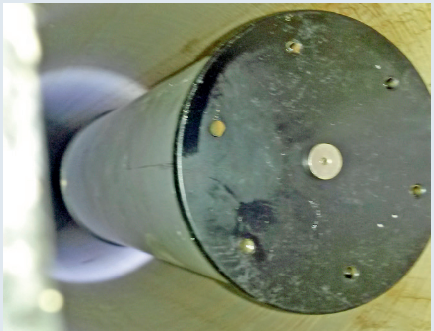
Figure 4: Pipe-Inspector® position at starting point
