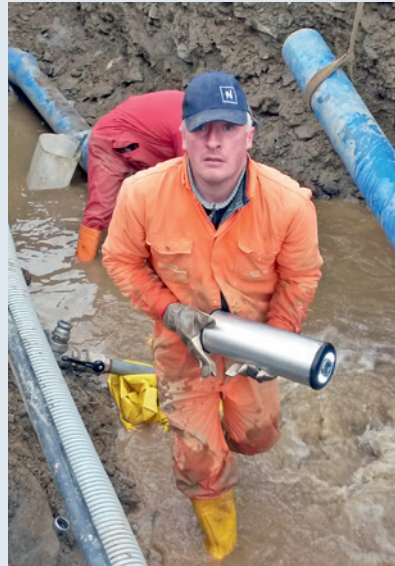
Figure 6: Pipe-Inspector® after retrieval
