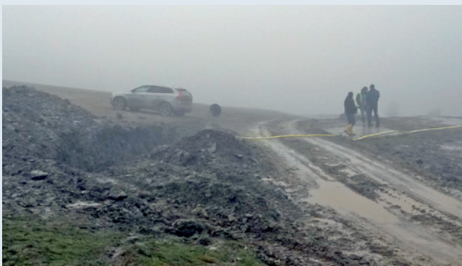
Figure 1: Site in over 2,000m above sea level
