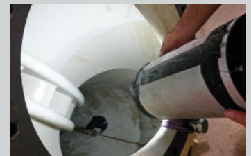
Removal at „Francis“ turbine
