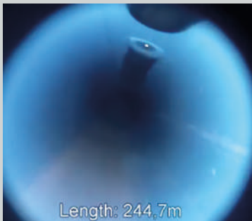
Drinking water pipeline inspection
