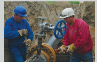
Insertion into gas pipeline
