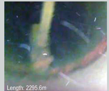
Length: 2295.6m Hydropower pipeline inspection: Foreign object „Hammer“
