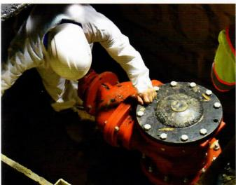
Start access sluice valve installed by DC Water forces
