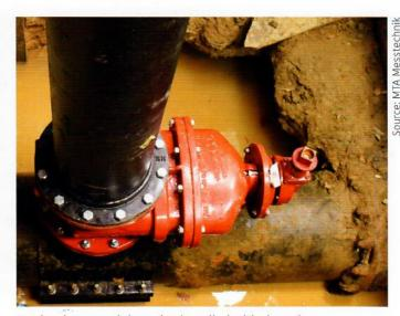
Retrieval access sluice valve installed with riser piece
