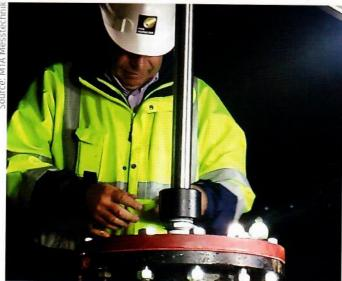
Plunging sleeve connection typical at both access points
