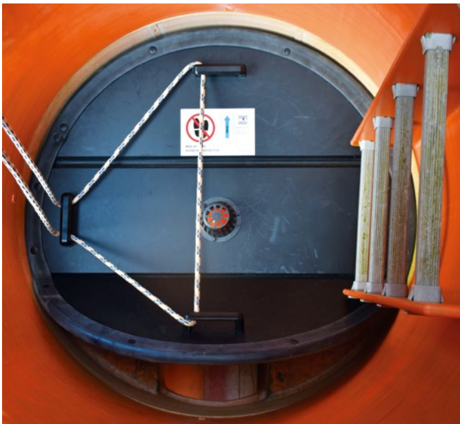
Adjust MTA SP 1000 in the manhole (pay attention to the flow direction - blue arrow on the sticker)
