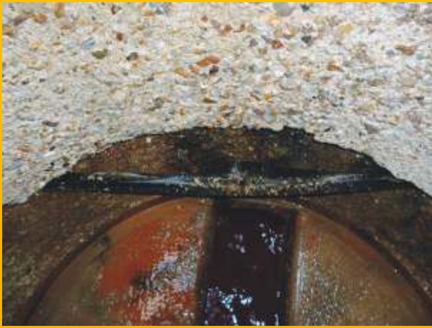
Concrete corrosion
