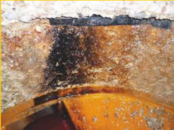
Concrete corrosion
